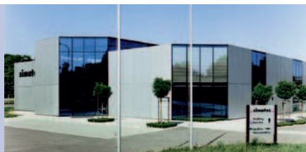
simatec ag, Wangen a.Aare, Switzerland
